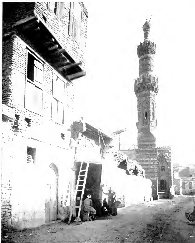
CAIRO, EGYPT. STREET WITH NO PAVEMENT.
